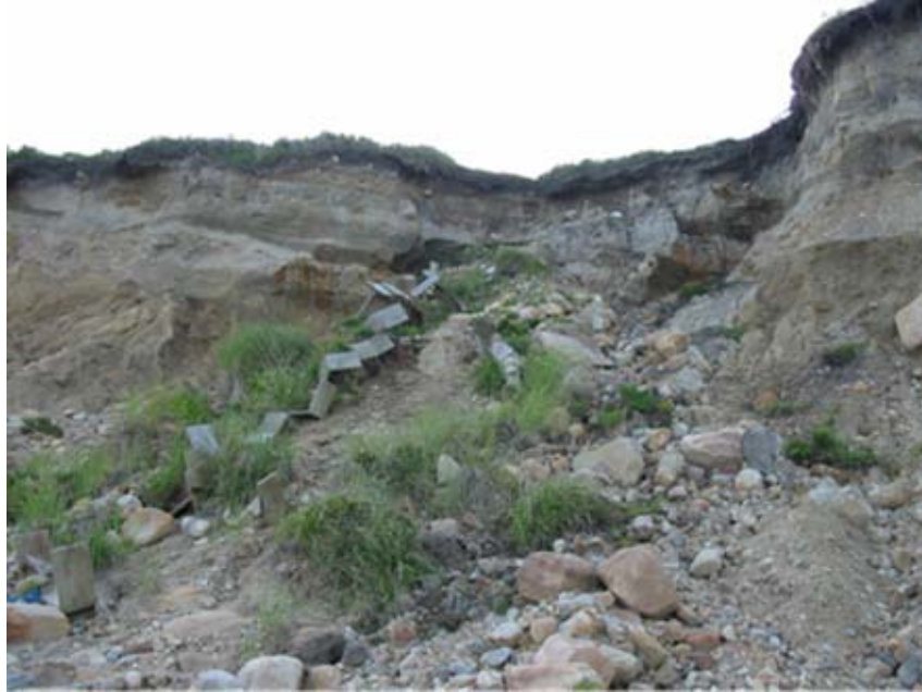
Figure 3. Photograph of mass wasting of the bluff face. The crest of the bluff recedes as material is transported down slope in the form of a debris slide. Remnants of terracing can be seen intertwined with boulders and gravel. Debris flows and slumps often carry vegetation as a coherent form.
