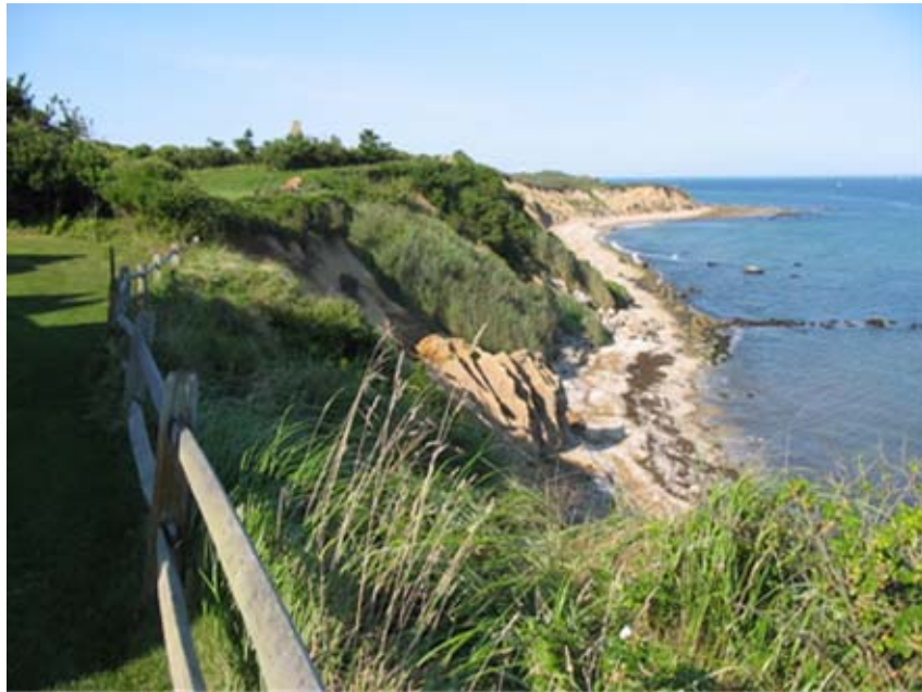
Figure 9. Slope reduction and vegetation appear to be the most effective stabilizing techniques. Regions of the coastal bluffs that have been stabilized with these mechanisms experience decreased recession
