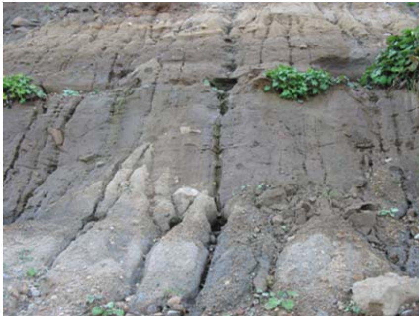
Figure 4. Groundwater seeping out of the face of the bluff where hardpan layers outcrop results in concentrated streams of water incise the face, dislodge material and undercut the clay lenses.
