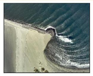
Figure 11. Mound diffraction structure as constructed at Grays Harbor, WA (2000)
