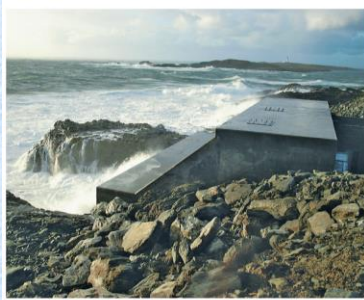
(a) Photo of the exterior of LIMPET 500, the world's first commercial wave power plant.
