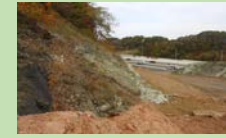
Cut road to be filled
