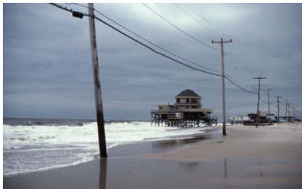
Aftermath of winter 1991 coastal storms at West Hampton Dunes.
