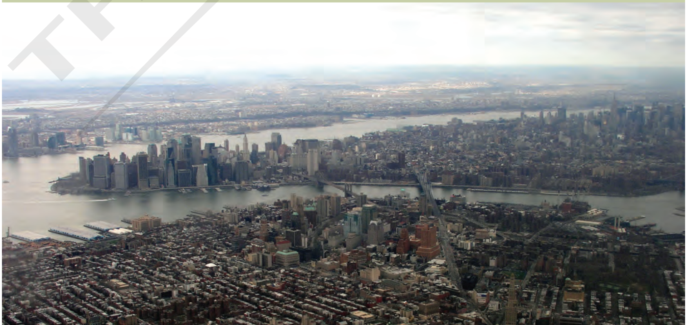
► Figure NY-NJ.27 Aerial view of the Manhattan skyline showing how building height is controlled by the subsurface geology. In the Financial District (left center) and Midtown (right of center), buildings are taller because they can be anchored in bedrock that is nearer the surface. In between, the buildings are shorter because the bedrock surface drops along faults, creating a valley that has been glaciated and filled with unconsolidated glacial sediments, which are not good for supporting tall buildings.
