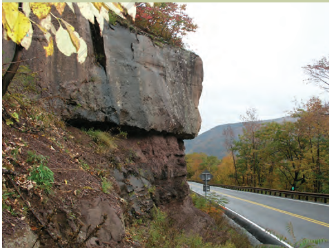
► Figure NY-NJ.3 High up in the Catskill Mountains, rock layers are horizontal, showing that the Catskill Mountains have been carved into the bedrock, which is relatively undisturbed. Road cut along NY Route 23A, near Palenville, New York.
